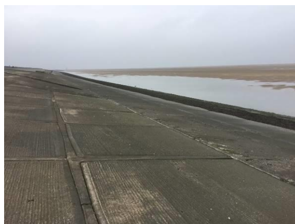
Figure 12: The Wallasey Embankment (Photo Source: CH2M Site Visit 29 th September 2017)
