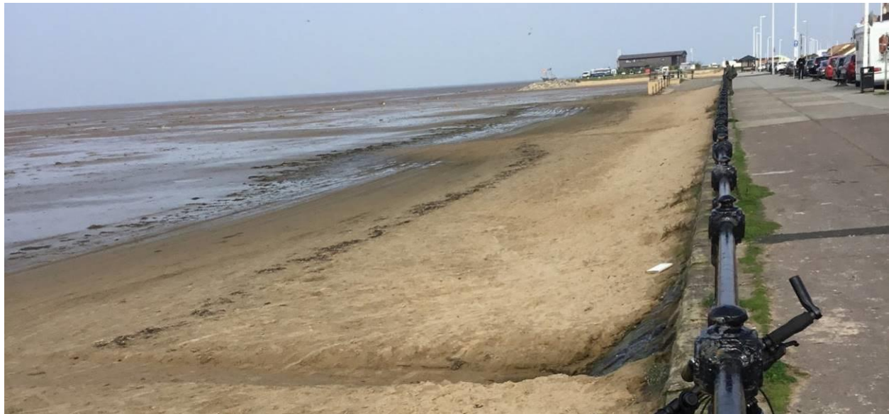
Figure 14: High beach levels next to the seawall at Hoylake (Photo Source: CH2M site visit 29 th September 2017)
